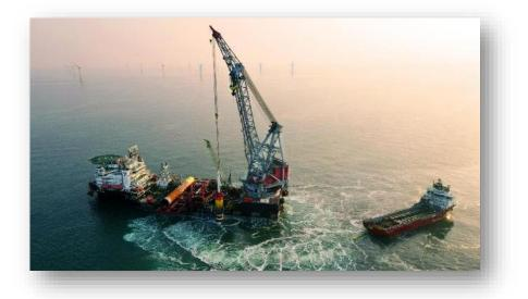
Figure 12 – Pile installation on DP
