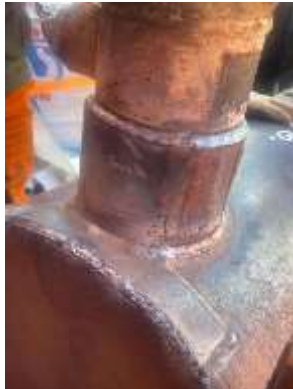
Sleeve welded at the area of corrosion.
