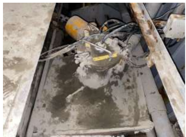
Temporary repairs with a cement box to restrict water leakage
