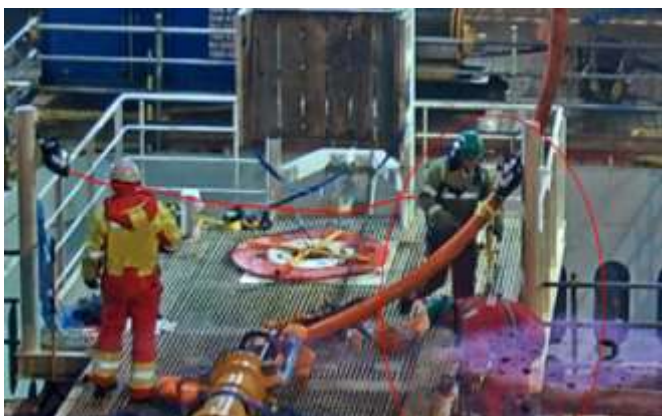
Showing person in green helmet before incident. His fall arrest line illustrated in red
