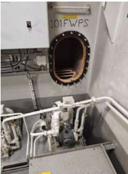
Entry to the tank viewed externally.
