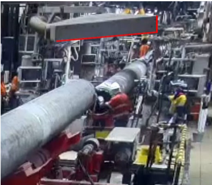
Extraction hood above firing line
