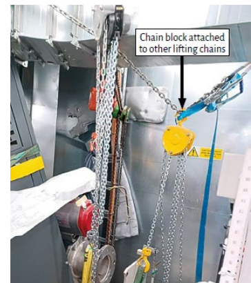
The lifting arrangements
