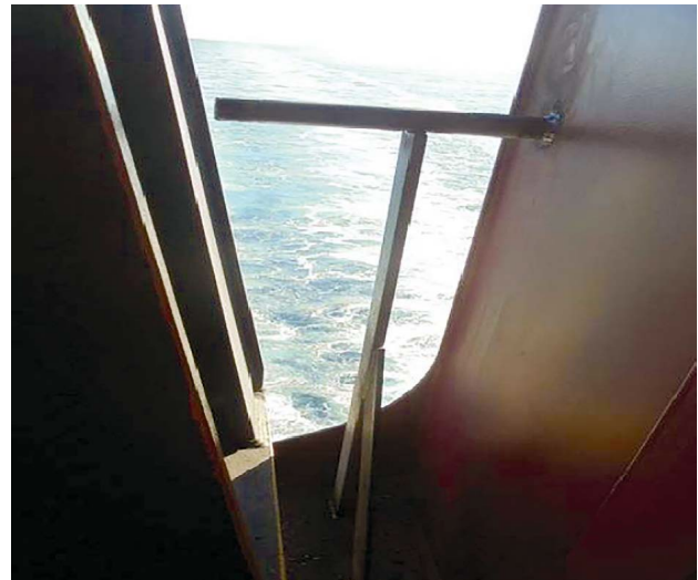
The guarded opening following remedial action
