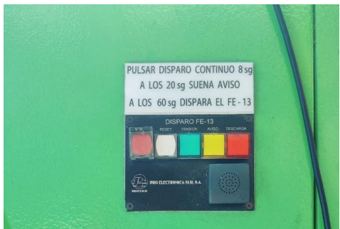
Firefighting dashboard (lefthand button with lid, activation button)
