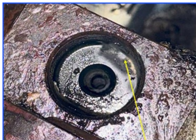
Pressure Fuel Pump Outlet Port Found With Sign Of Fuel Leakage
