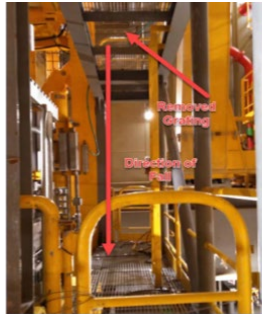
Hatch cover removed
