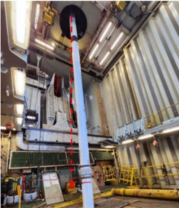
Workstation showing dropped impact point
